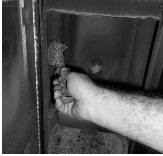
Figure 48 - Cleaning the interior
