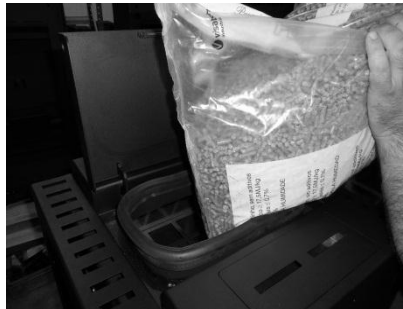
Figure 42 - Refilling the pellet reservoir
