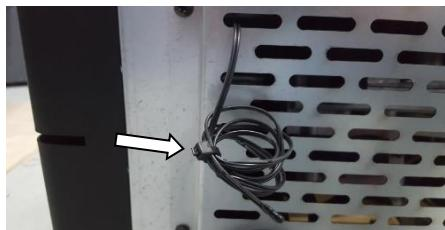
Figure 9 - Room temperature probe
