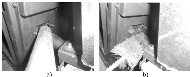
Figure 109 - a) Vacuum the interior; b) Clean using a brush
