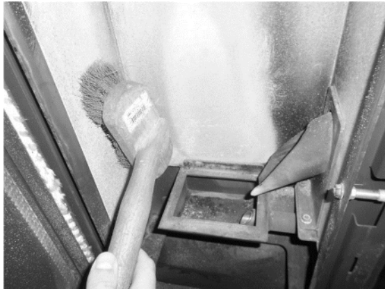
Figure 106 - Cleaning the vermiculite
