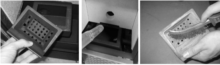
a) Burner removal
