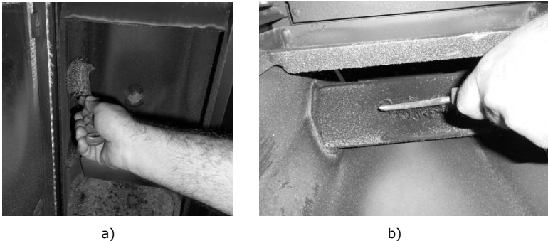
Figure 31 - Cleaning the interior of the backboiler model
