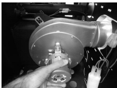
Figure 42 - a) Remove the screws; b) Remove the extractor
