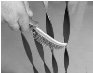
Figure 41 - Cleaning the air flow pipes and turbulators
