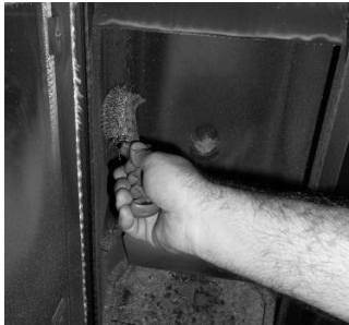
Figure 26 - Cleaning the inside of the water compact
