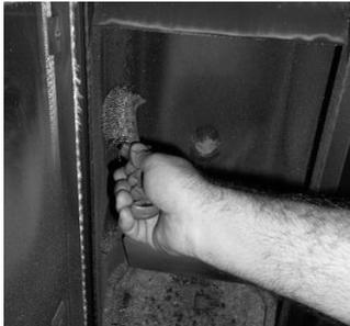
**Figure 26 - Cleaning the inside of the water compact**
