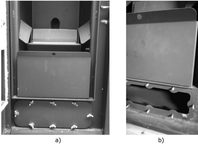
**Figure 32 - Cleaning the inside of the compact**
