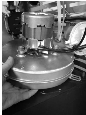
Figure 34 - a) Remove the screws; b) Remove the extractor
